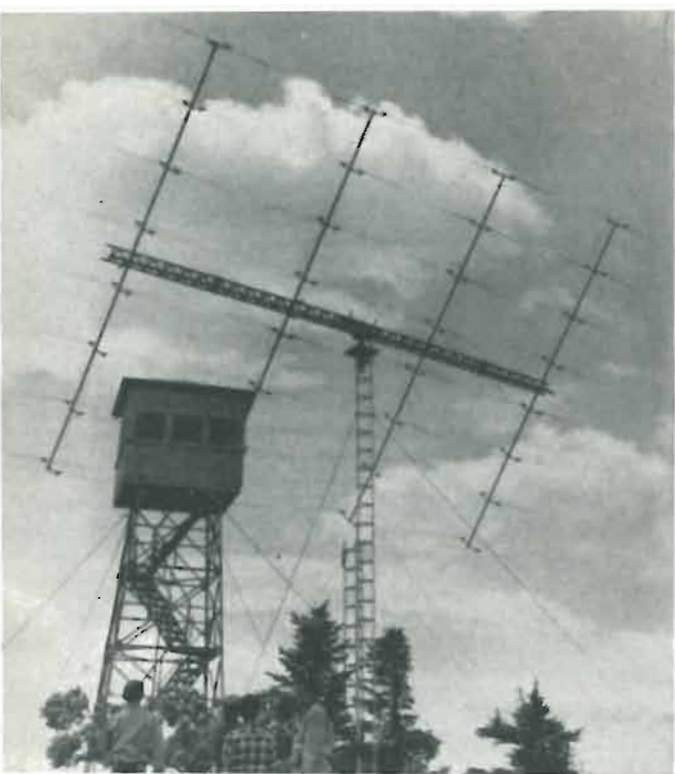
Incentive licensing may stimulate experimental work by American hams, like this antenna and moon-bounce communications installation operating on 144 MHz.
